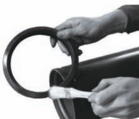
Lubricate gasket
