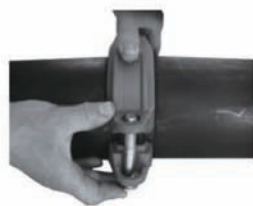
Housing installation
