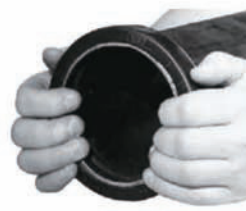
Gasket installation
