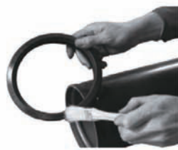
Lubricate gasket
